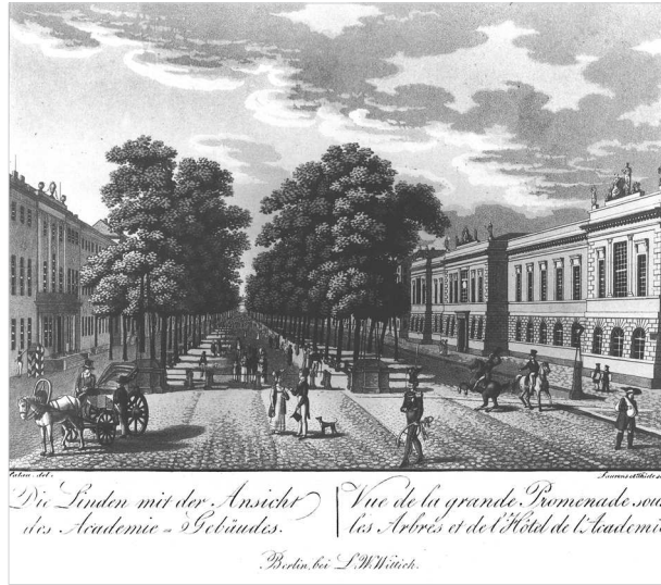
Figure 7. The academy building on Unter den Linden , its location from 1752 to 1904; drawing by Calau, engraving by Lauréns and Thiele.
